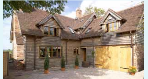
SPOT THE BOREHOLE: THIS HOME BY OAKWRIGHTS USES GROUND SOURCE HEATING WITH BOREHOLES CONCEALED UNDER THE DRIVEWAY
